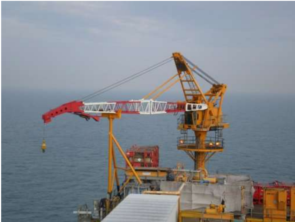
Pedestal lattice boom crane.
